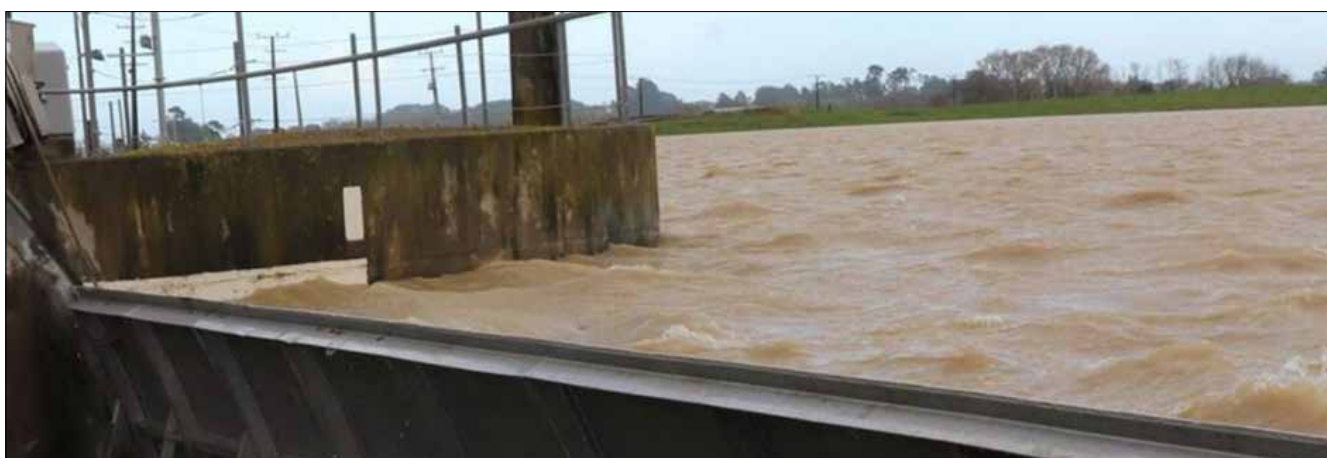
The Manawātū River in flood. The floodgates can be opened slowly and strategically from the bottom up to release water from the river into the spillway when water reaches a critical height.
